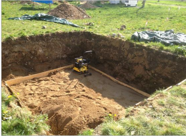
Figure 4.3. Compaction of soil at 1 m depth with a vibratory plate compactor.
