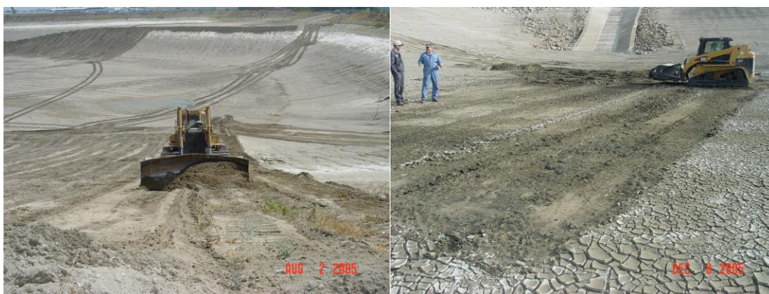
Figure 2.9. Scraping of the top layer of clogged infiltration basins in the USA. Source: Hutchinson et al. (2018)
