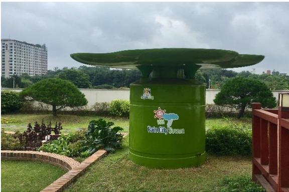
**Figure 7.1** Small-scale rainwater facility (rainwater storing pergola installed on the rooftop of the Suwon City Hall)
