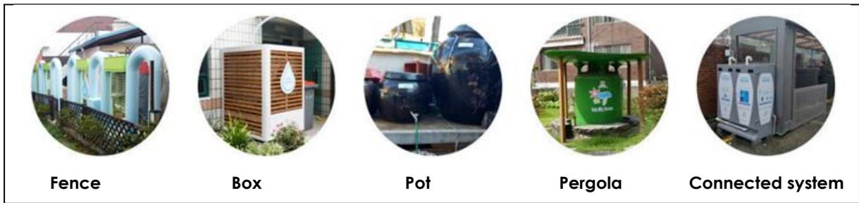
**Figure 7.18** Types of small-scale rainwater storage (Source: SG, 2018)
