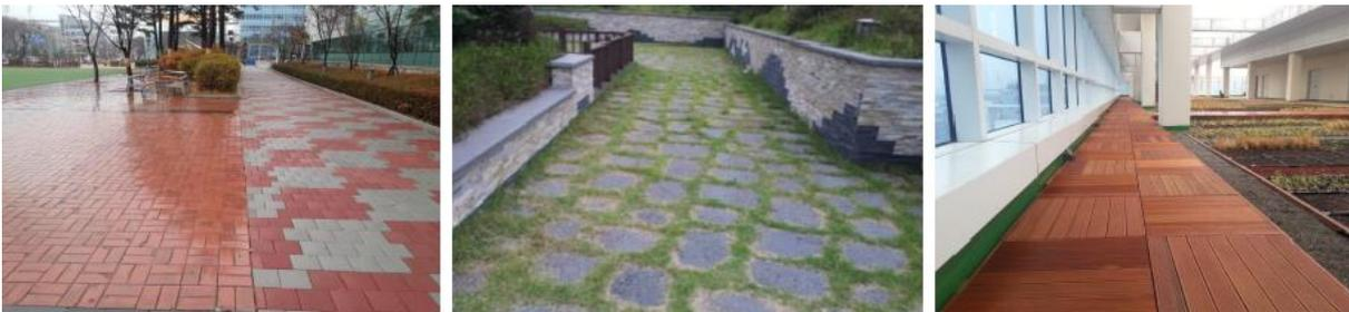
**Figure 7.19** Permeable pavements (blocks) in Jangan district office (Source: SG, 2014)
