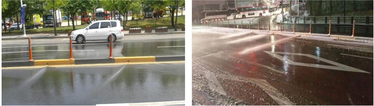
**Figure 7.21** Road sprinkling system using rainwater (left) and liquid de-icing material (right)
