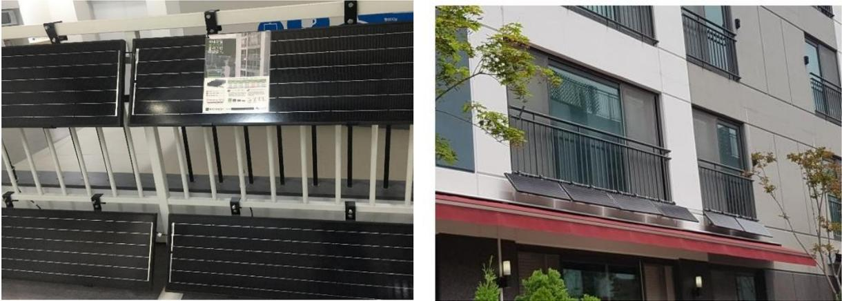
**Figure 8.1** Small-scale solar energy generator installed on the veranda rail in two rows (left) and between floors (right)
