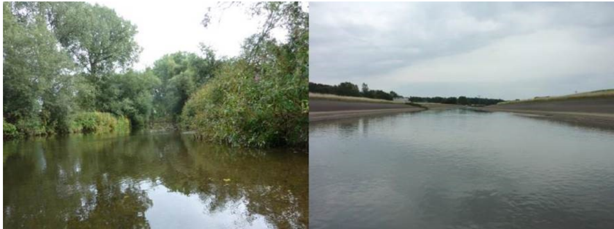
FIGURE 2.1. STUDY REACHES IN JULY 2015. NATURE (LEFT) WAS UN-ALTERED, AND FEATURED A MEANDERING PATTERN WITH POOLS AND RIFFLES. CHANNEL (RIGHT) WAS STRAIGHTENED AND CONCRETE LINED.
