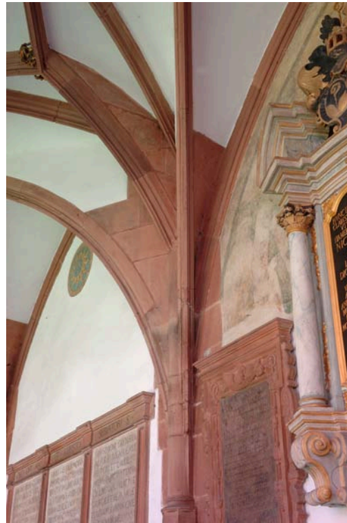
Fig. 8: Ploughshare webs in the vault of the cloister in Basel Minster, c. 1465 (A. Kobe).
