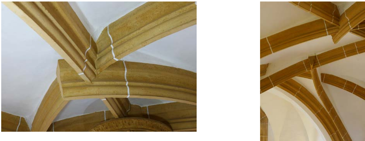
Fig. 5: Details of the rib system. Left, keystones with triple intersection near the summit. Right, the gap between the curvilinear ribs, showing that their course is discontinuous in the third dimension (M.J. Ventas Sierra / D. Wendland).
