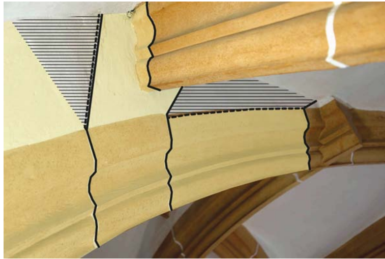
Fig. 9: Detail of the stone members of the vault in the “Hall of Arms”. For clarity, the stone surfaces are highlighted, plastered portions marked as hatched areas, and the joints retraced (A. Kobe).
